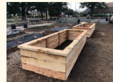
Volunteers work on constructing the garden beds
